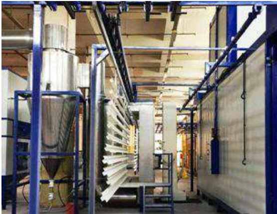
• BAR TRANSFER AUTOMATIC SYSTEMS
